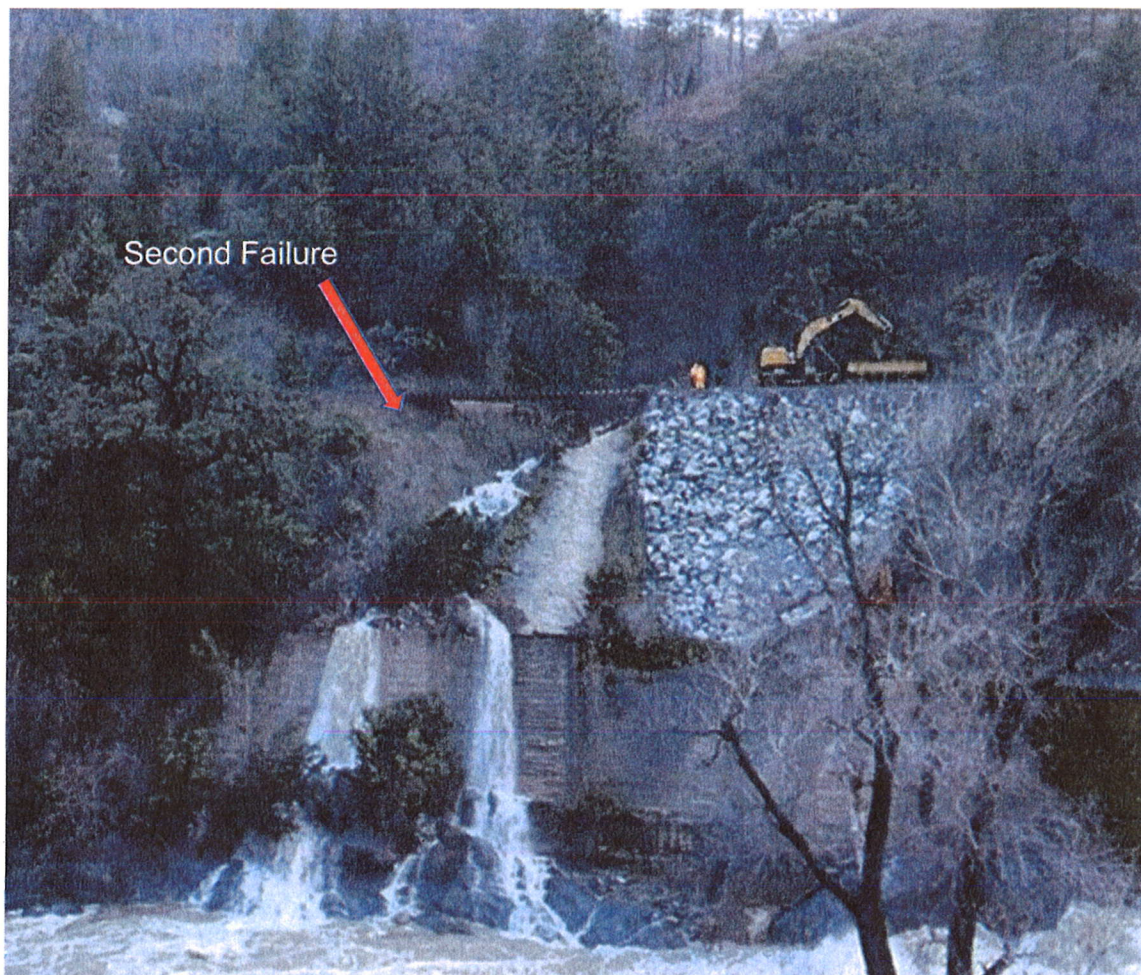
Image 4: January 12th, 2017. Complete washout of the railbed.
