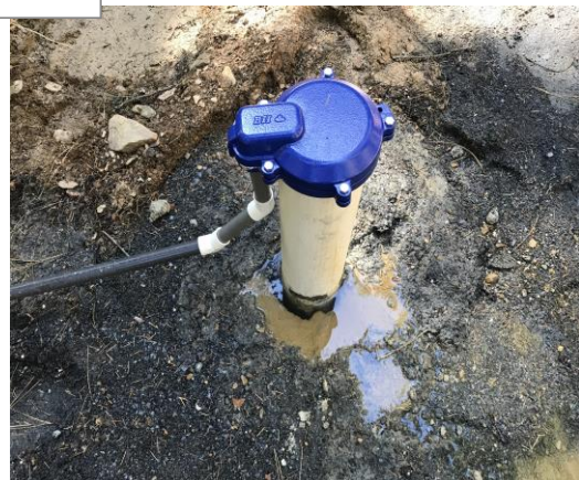
Newly Constructed Domestic Well near Quincy
