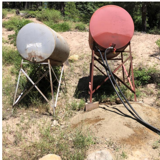
Poorly managed ASTs. These tanks have since been relocated and the spill hazards mitigated.
