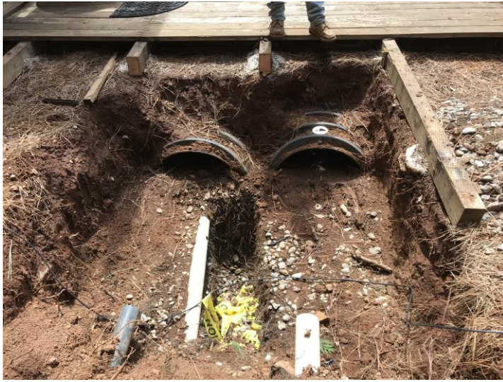
Root-clogged Onsite Wastewater Treatment System near Lake Almanor
