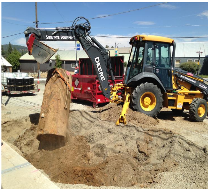
Underground Tank Removal, Pacific Street Portola
