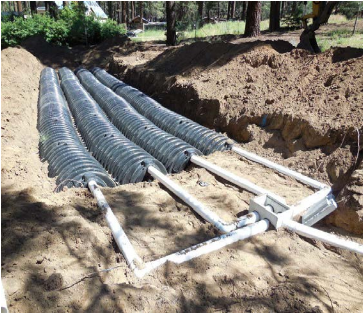
Gravel-less Onsite Wastewater Treatment System off Grizzly Road near Beckwourth
