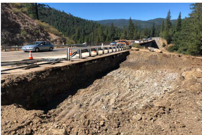
Contaminated Soil Removal at Spanish Creek Bridge, September 2018
