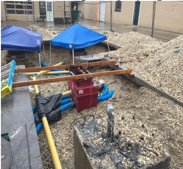
Underground Piping repair at One Stop Gas Station, Quincy
