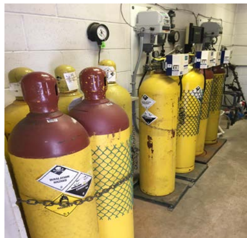
Chemical injection system, wastewater treatment plant Chester Public Utilities District
