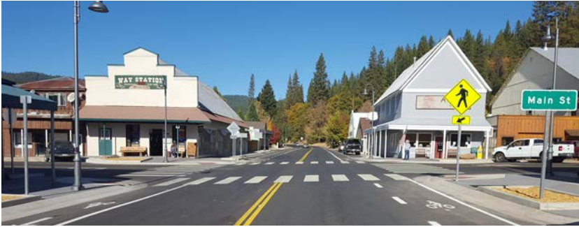
Figure 2-22: After State Route 89 Rehabilitation Project showing marked crosswalks and bike lanes at SR 89 and Main Street in Greenville
