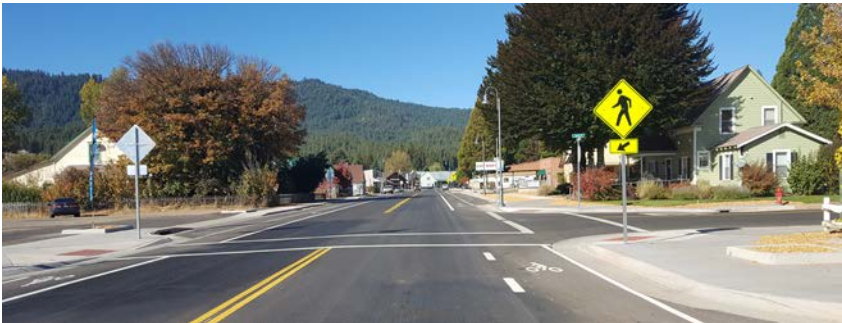
Figure 2-24: After State Route 89 Rehabilitation Project at SR 89 and Jessie Street showing new sidewalks and bike lanes
