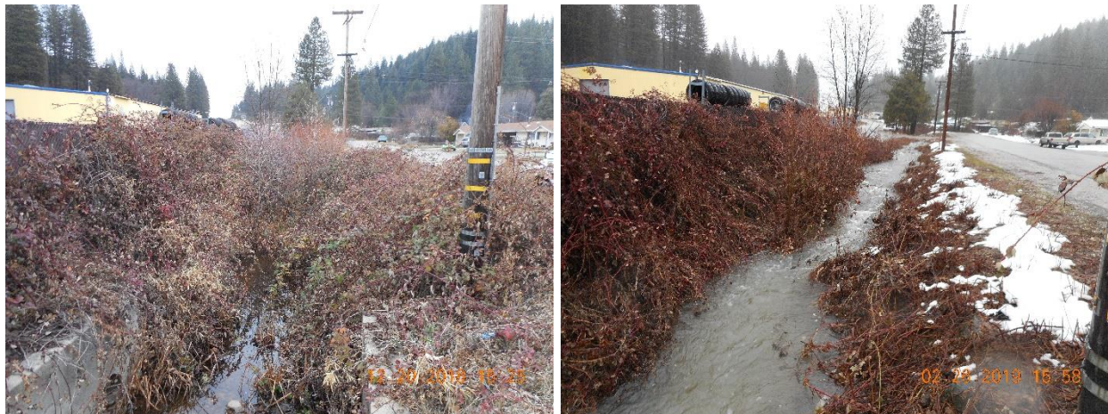
Figure 2-1 Vegetation Removal behind Les Schwab Tire – Before and After
