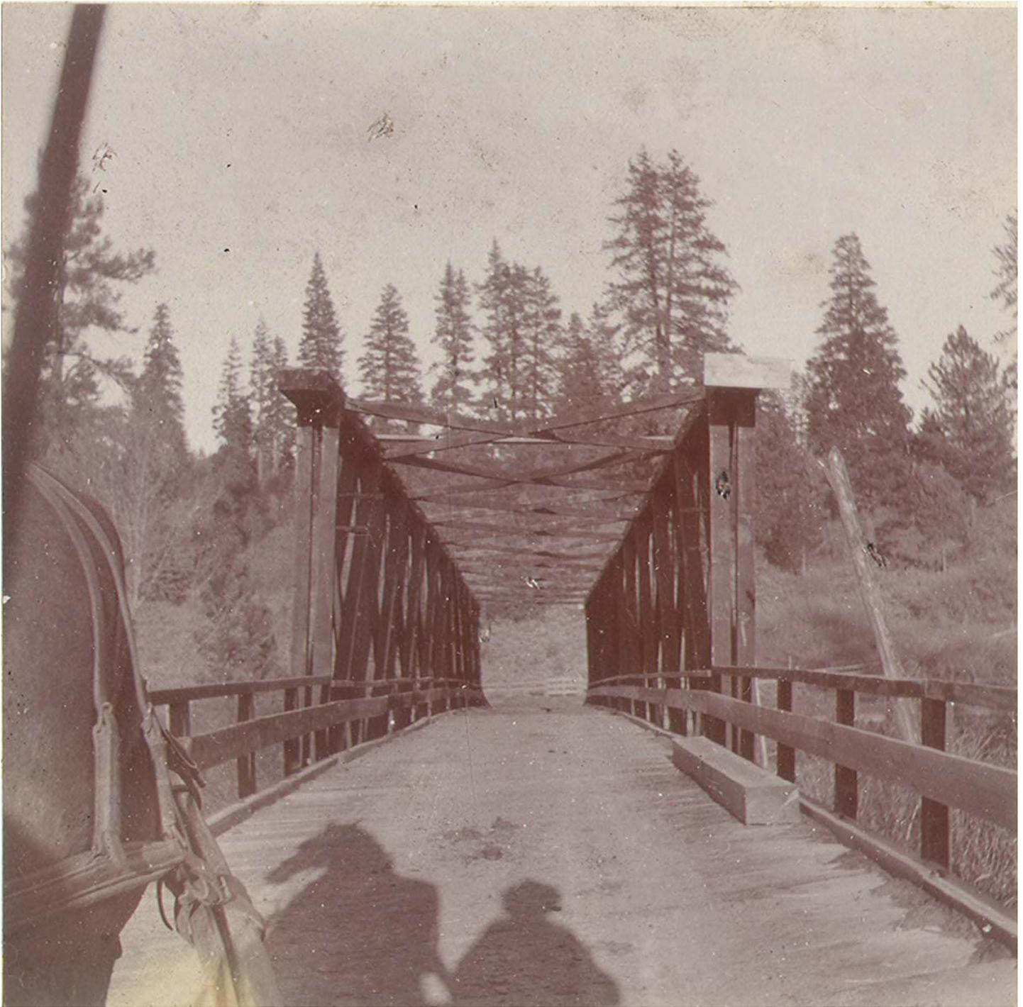
***The Mohawk Howe Truss Bridge at the Denten Place in the 1890s. In 1902, it was replaced with the current steel structure. Neither bridge at this site was ever washed out in floods. View is to the east from the Graeagle side of the Middle Fork Feather River.***
