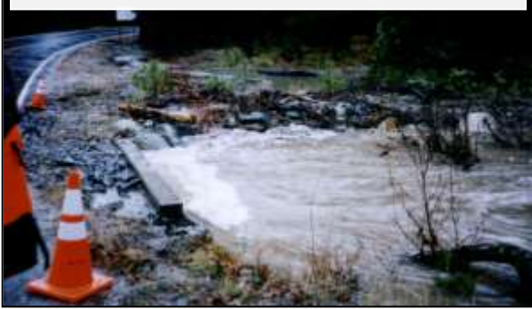
Barry Creek @ Hwy. 89 culvert, December 31, 2005
